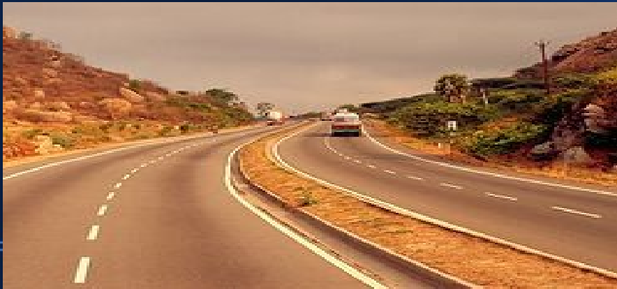
A section of the Golden Quadrilateral highway from Chennai – Mumbai phase
